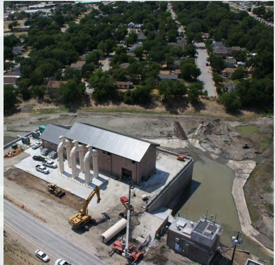
2012 New Pavaho Pump Station
