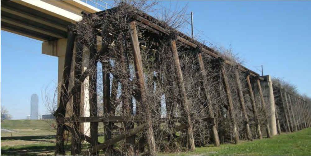
Old abandoned AT&SF Trestles Proposed for Removal
